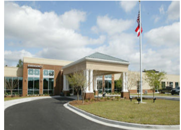
Clinch Memorial Hospital Homerville, GA
